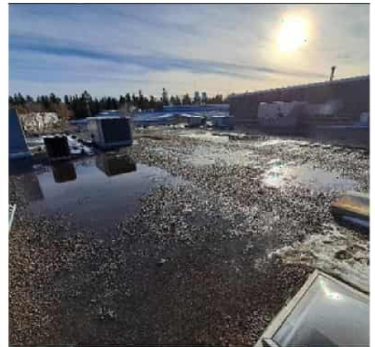
Meltwater on Jan 30th. All of this water has to either evaporate or drip through the roof. As you can see it is not draining very well.
